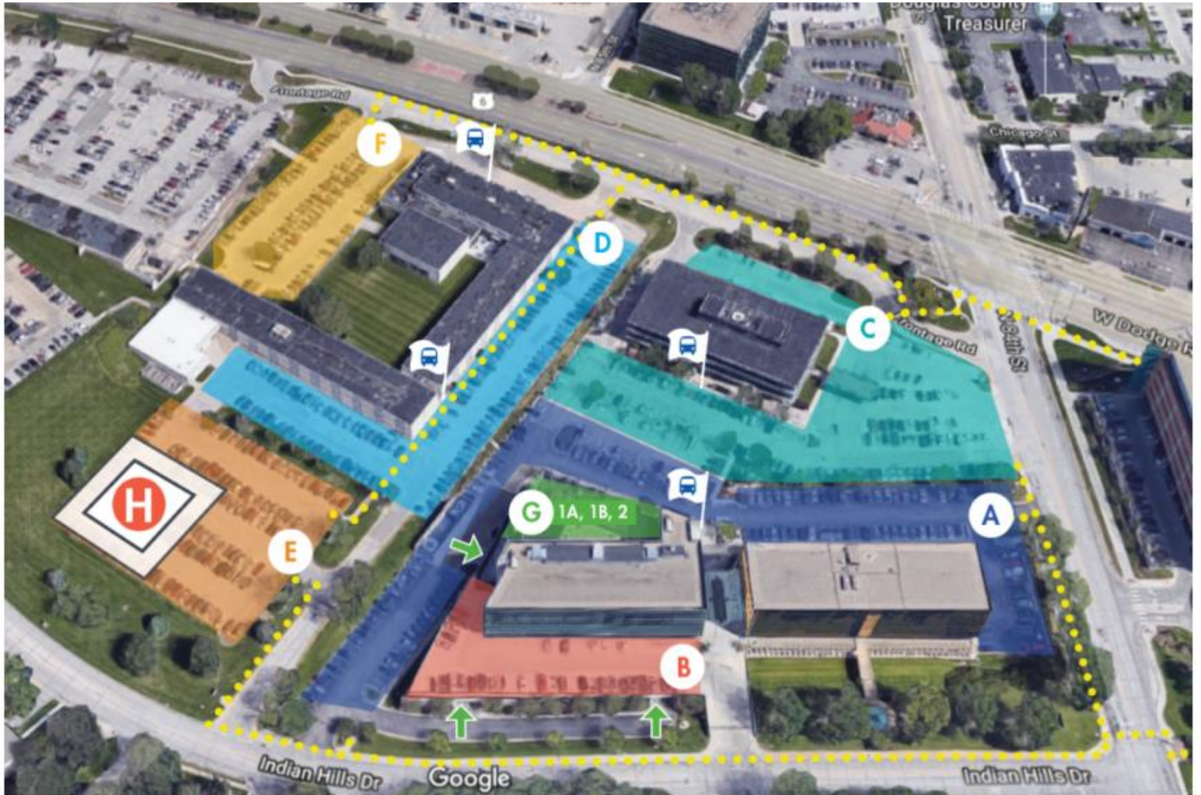
The "H" circled in orange indicates where a temporary helipad is under construction in Indian Hills parking Lot E.
